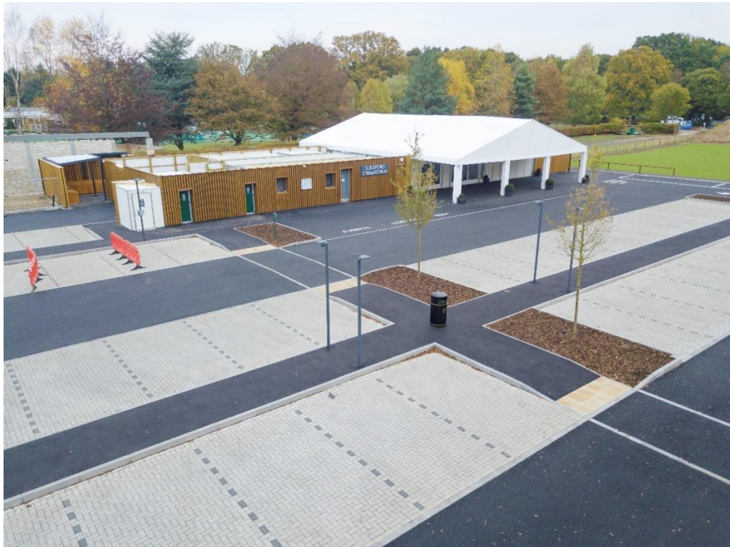
Photo 4: External view of Temporary Chapel (Credit Dan Hannington)
