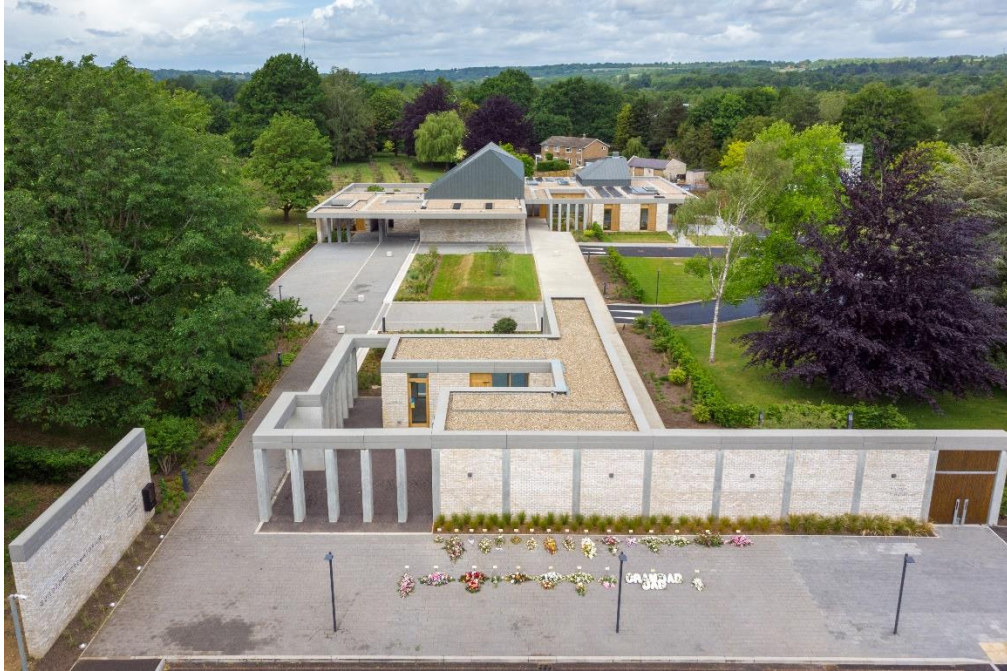
Photo 9: View of completed project (Credit Dan Hannington)
