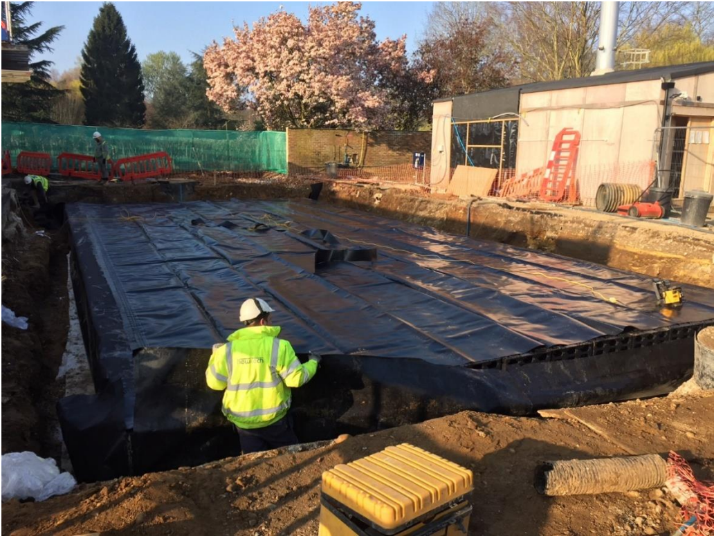
Photo 2: Part of SUDs system being installed
