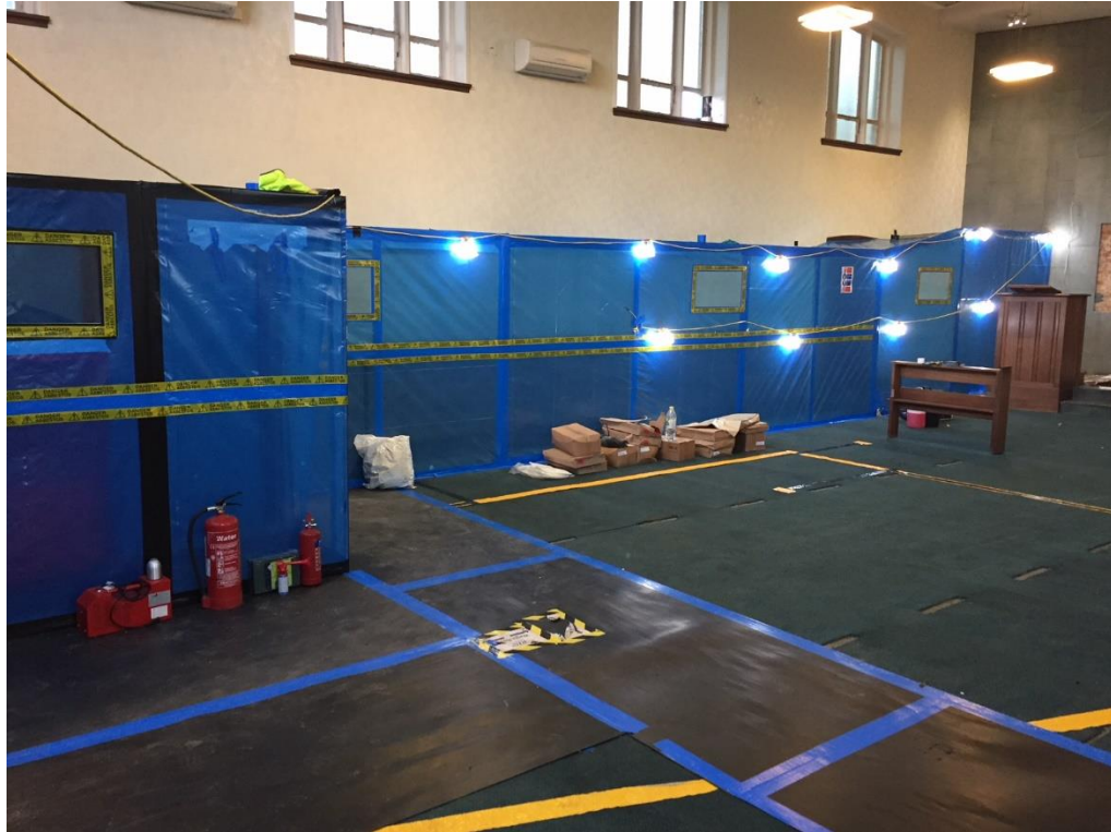
Photo 6: Preparation for removal of concealed asbestos
