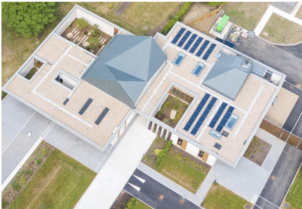
Photo 3: PV array on roof of new building (Credit Dan Hannington)
