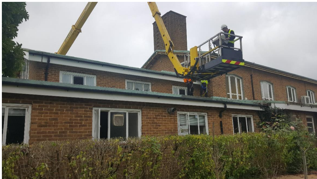
Photo 7: Removal of bat roosts being undertaken by hand under supervision of an ecologist and in accordance with EPSL.
